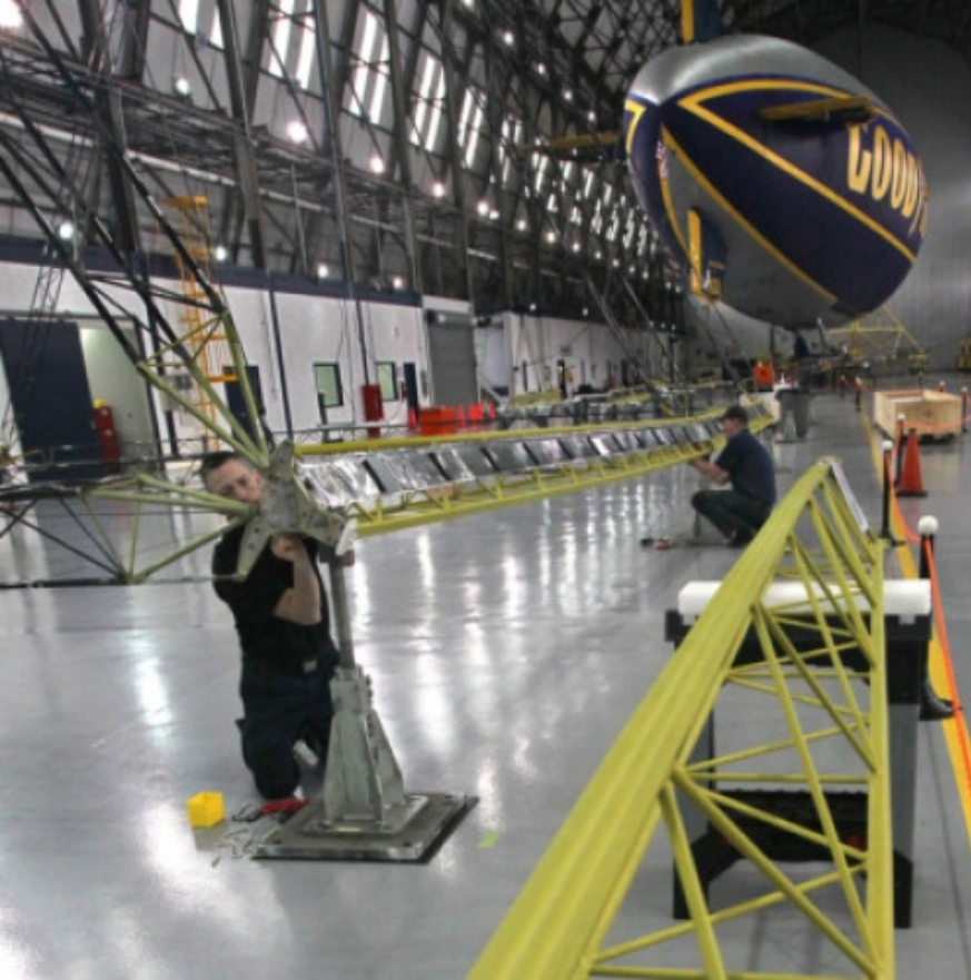
Goodyear airship mechanic Tom Bradley (left) and Marcus Draeger, an airship mechanic with the German Zeppelin Corporation, work on a section of the interior frame as construction of the first of Goodyear's new fleet of airships, the Goodyear NT, begins at the Wingfoot Lake hangar on Friday, in Suffield Township. The Spirit of Goodyear blimp is in the background.
