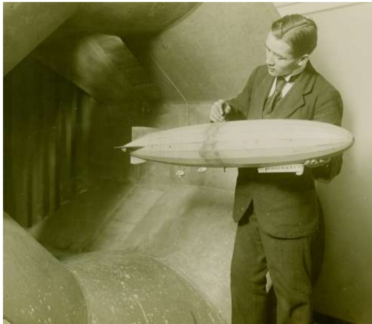
Model of LZ-120 in Göttingen wind tunnel – ca. 1920
