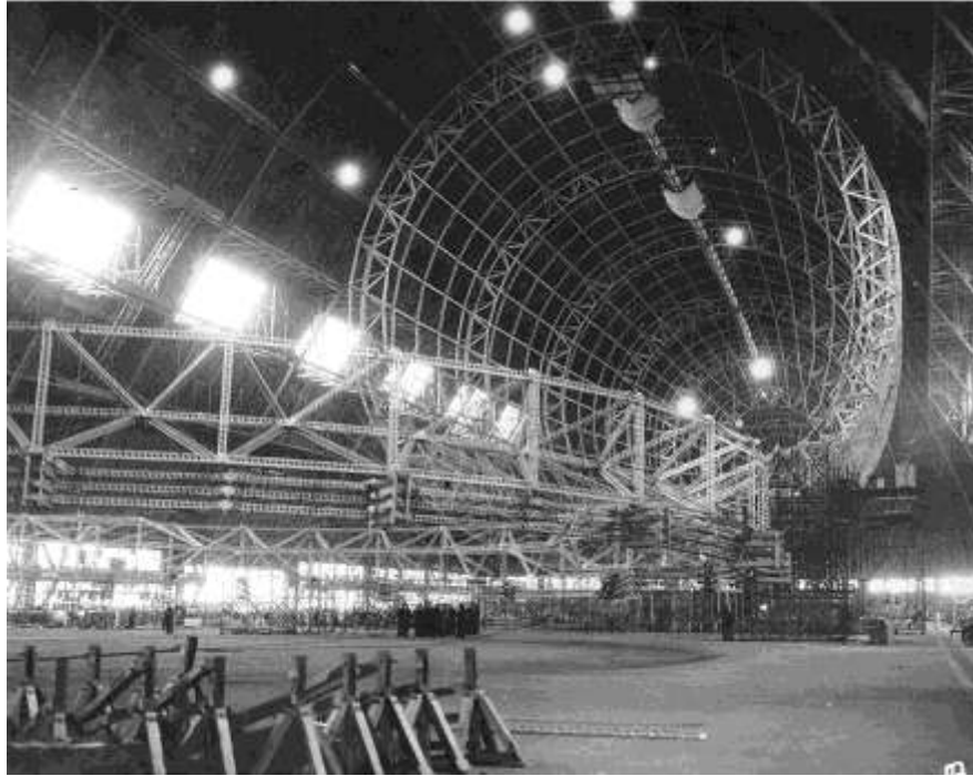
Erection of rings to form hull of the USS Macon
