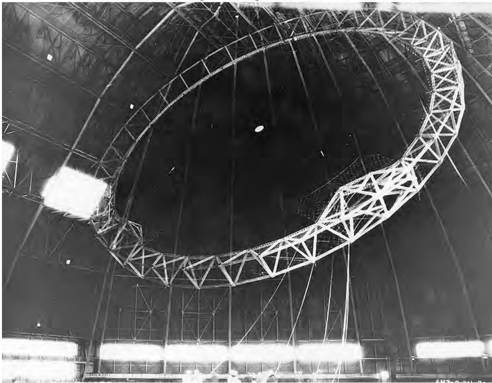
Photo # NH 43121 Erecting the first ring of USS Akron's frame, March 1930
