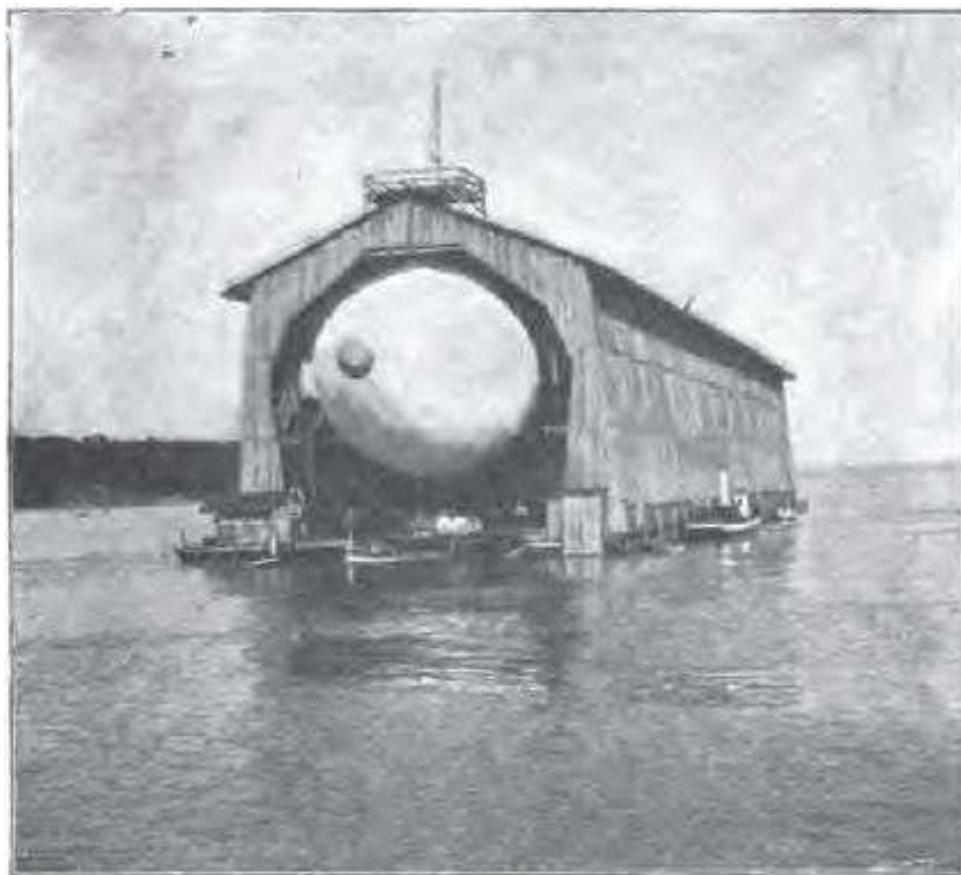
The Luftschiff Zeppelin 1 (LZ-1) in its floating hangar on Lake Constance (Bodensee), near Friedrichshafen
