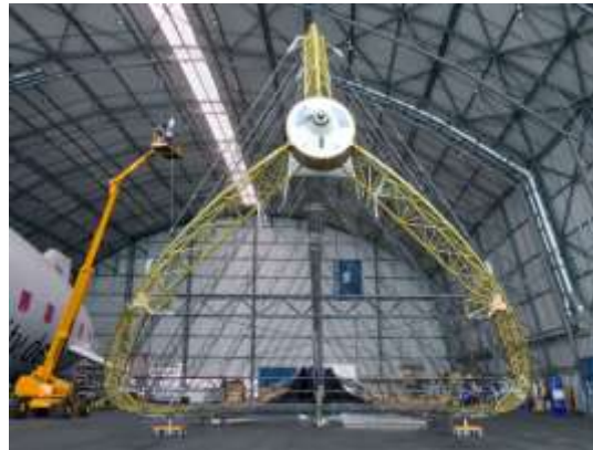
Erection of Framework
