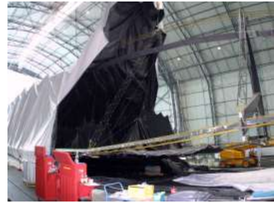
Slipping the Hull over the Frame
