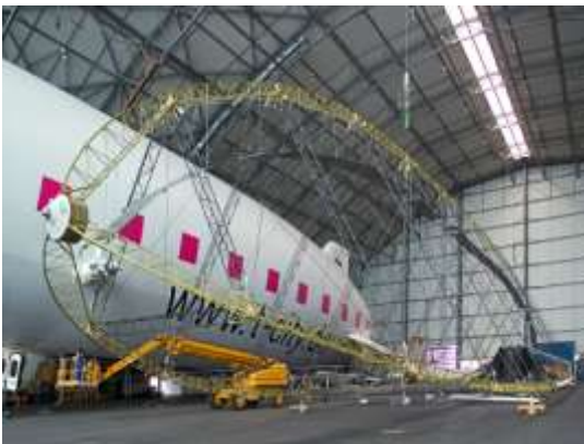
Erection of Framework
