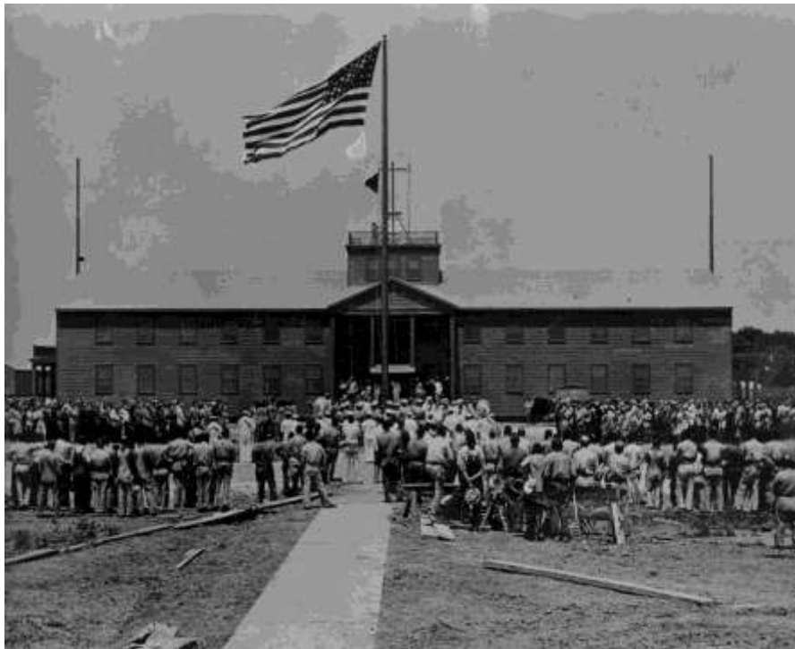
The Non-Commissioned Officers' barracks of the Houma Naval Air Station during construction.
