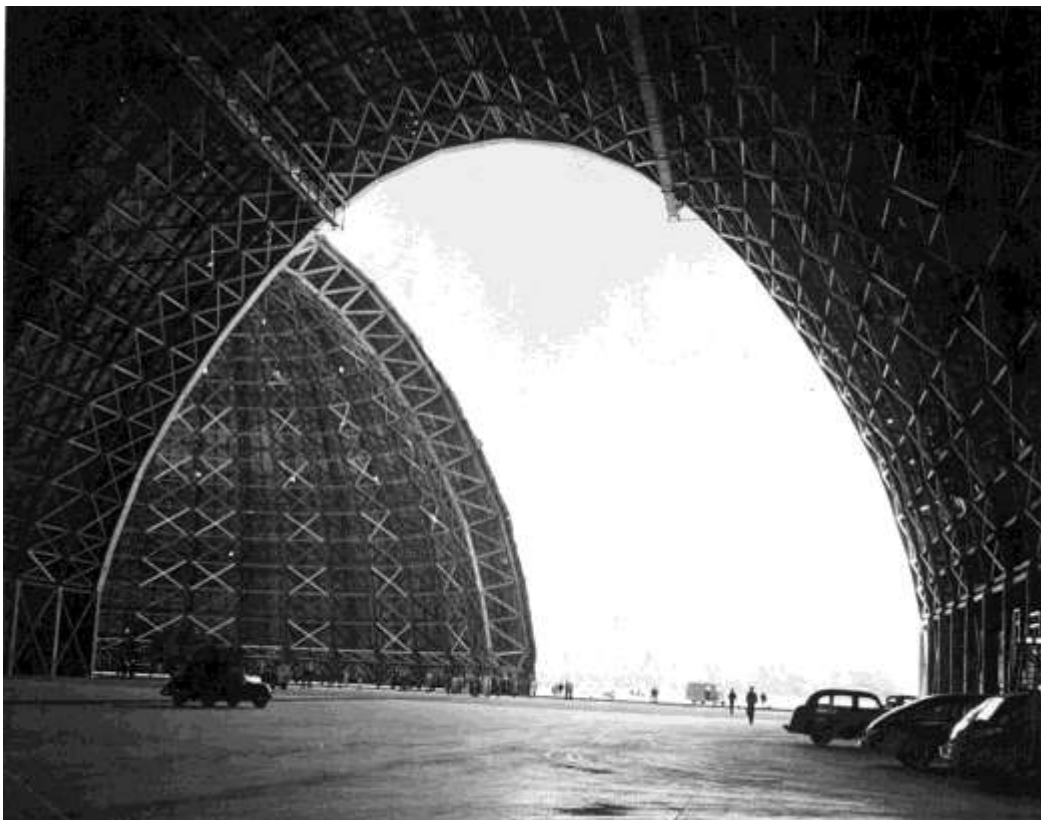
An interior view of the blimp hangar at the Houma Naval Air Station. The cars and people give some idea of scale.
