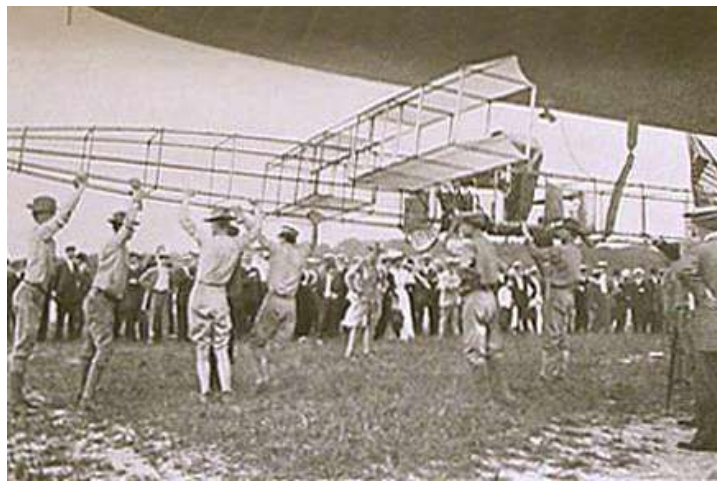
Baldwin Airship: SC-1 being moved at Fort Meyer.
